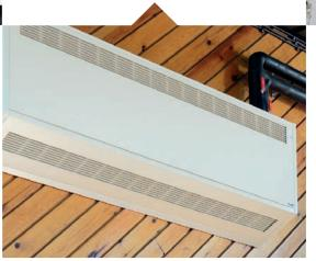
The second stage of our work saw us retrofit a fan coil heating system in the school's main hall, embedded in the walls.
